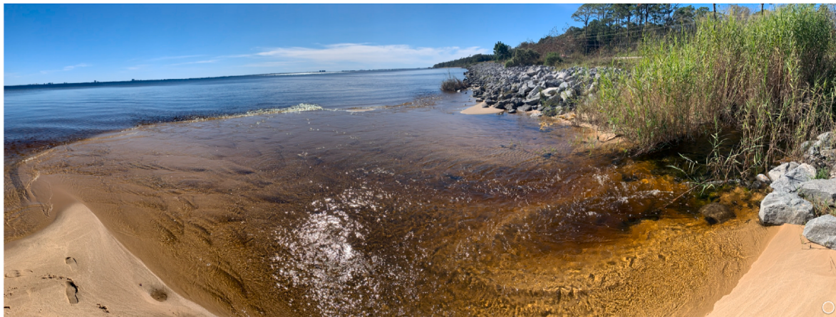
Fig. 2. Deteriorating riprap revetment (right) near a culvert along FL-20 in Freeport, FL that is cause of concern for a deteriorating section of FL-20. Such conventional infrastructure is a prime candidate for enhancement during repair to restore its primary engineering function while broadening the biodiversity and other benefits associated with the structure (Photo Credit: M. Bilskie).
